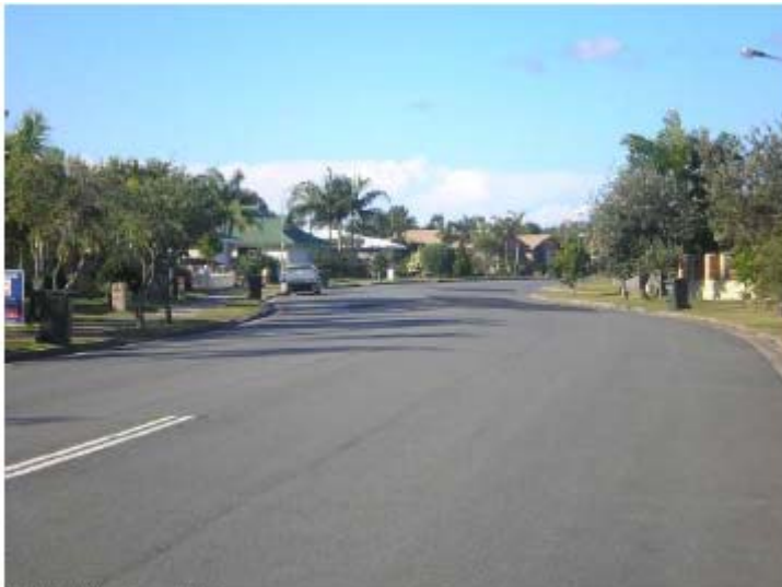
Residential Streetscape: Existing
