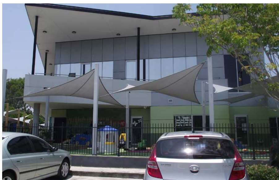
Figure 7.1 - Child care and service facilities - The incorporation of childcare and other service facilities within a business development increases its desirability for employees and contributes to the overall diversity of land uses. The siting of childcare facilities needs to be carefully considered against other business development uses, particularly relating to noise, vibration, security and potential hazardous land uses.
