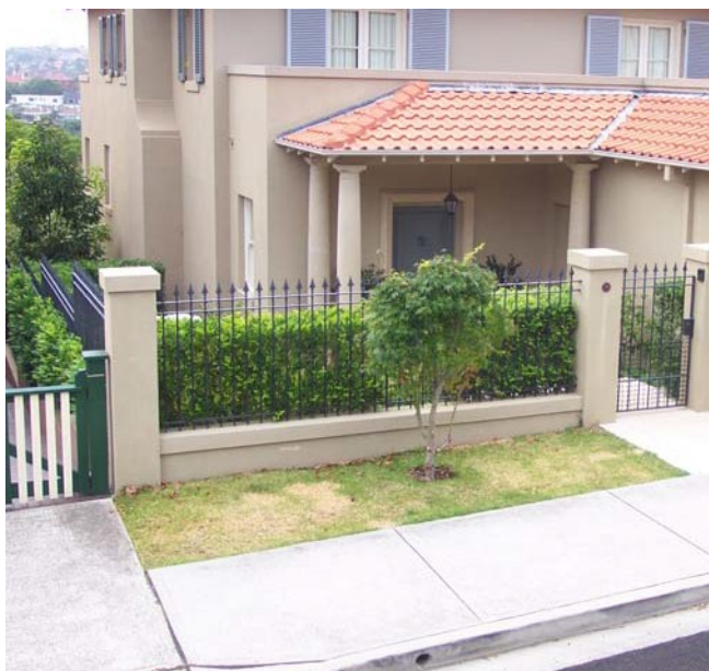
This fence returns down the side boundary, combines landscaping, open fencing and low walls to create a fence that enhances the pedestrian scale and residential qualities of the street.
