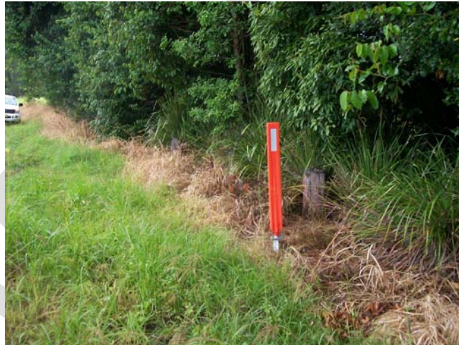
Figure 4 - HCV roadside marker post
