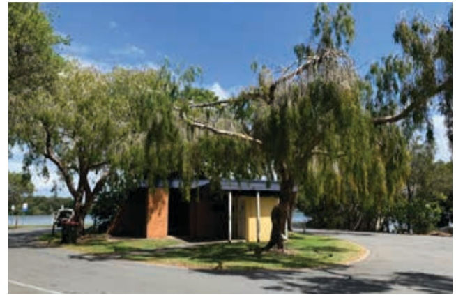
John Oxley Park at Chinderah will be upgraded after it was damaged by floodwaters in 2022.
