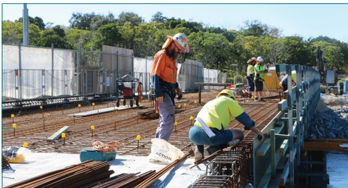
Workers steeling the deck of the new traffic bridge.
