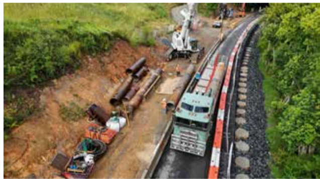
Demobilising crane and piling rig at Tyalgum Road slip site.
