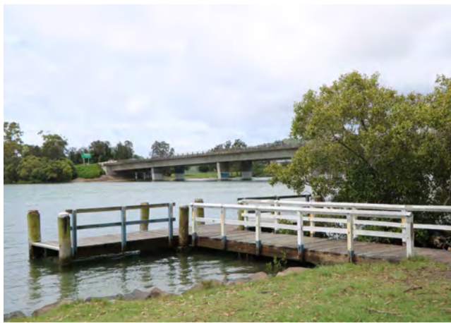
The old jetty at Dry Dock boat ramp will be removed and replaced with a new pontoon.
