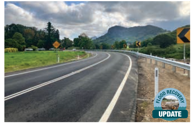
Recently completed flood restoration works at Kyogle Road.
