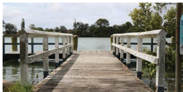
Dry Dock Road boat ramp is set to undergo an upgrade in 2025, making it safer and welcoming for people of all abilities.
