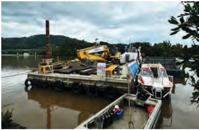
Barge-based maintenance being carried out on Tweed drains.
