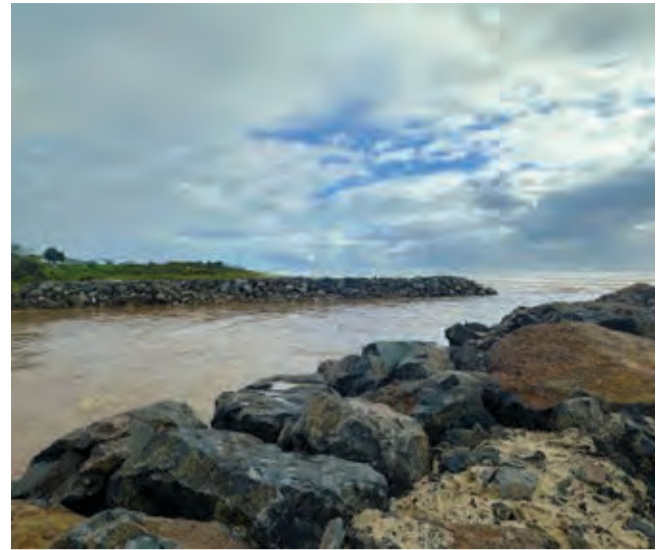
Mooball Creek seawalls after restoration works were completed.
