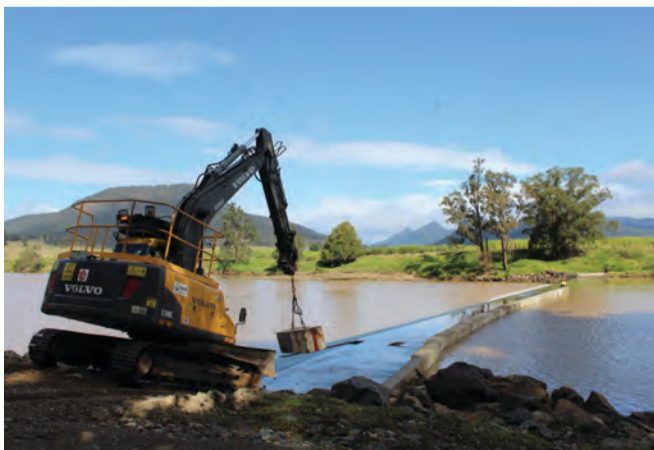
Cement blocks being placed at Bray Park Weir.
