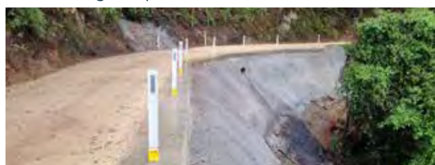
Works have been completed early on Cudgera Creek Road.
