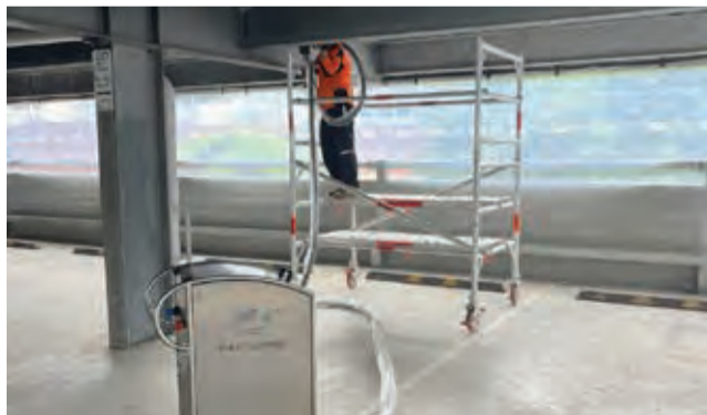
Worker on site at the multi-level carpark in Murwillumbah.
