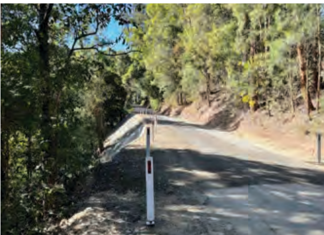
Completed road works at Pinnacle Road, Pumpenbil.
