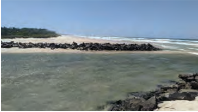
Mooball Creek seawall restoration will begin later this month.
