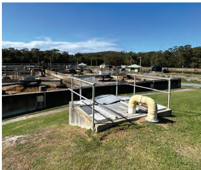
Hastings Point Wastewater Treatment Plant.
