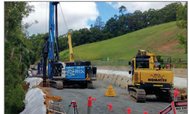
Work is underway on Tyalgum Road.
