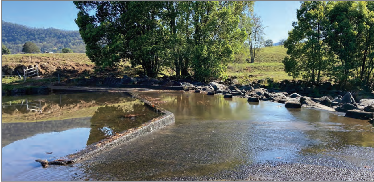
The Tyalgum Weir on the Oxley River is where Council sources water for Tyalgum. The river flow has reduced and the weir pool has dropped to the level that triggers Level 2 water restrictions for the village.
