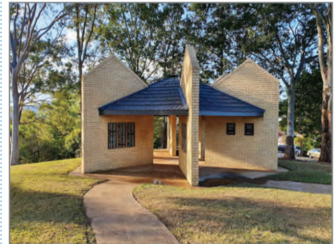
Restoration works at Murwillumbah's Banner Street Memorial Park have been completed.
