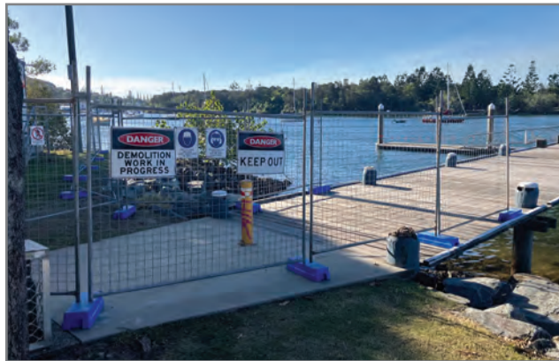
Rehabilitation works on Foysters Jetty is currently underway.
