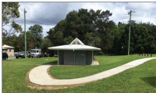
The public toilet in the park at Burringbar Memorial Reserve is being upgraded.
