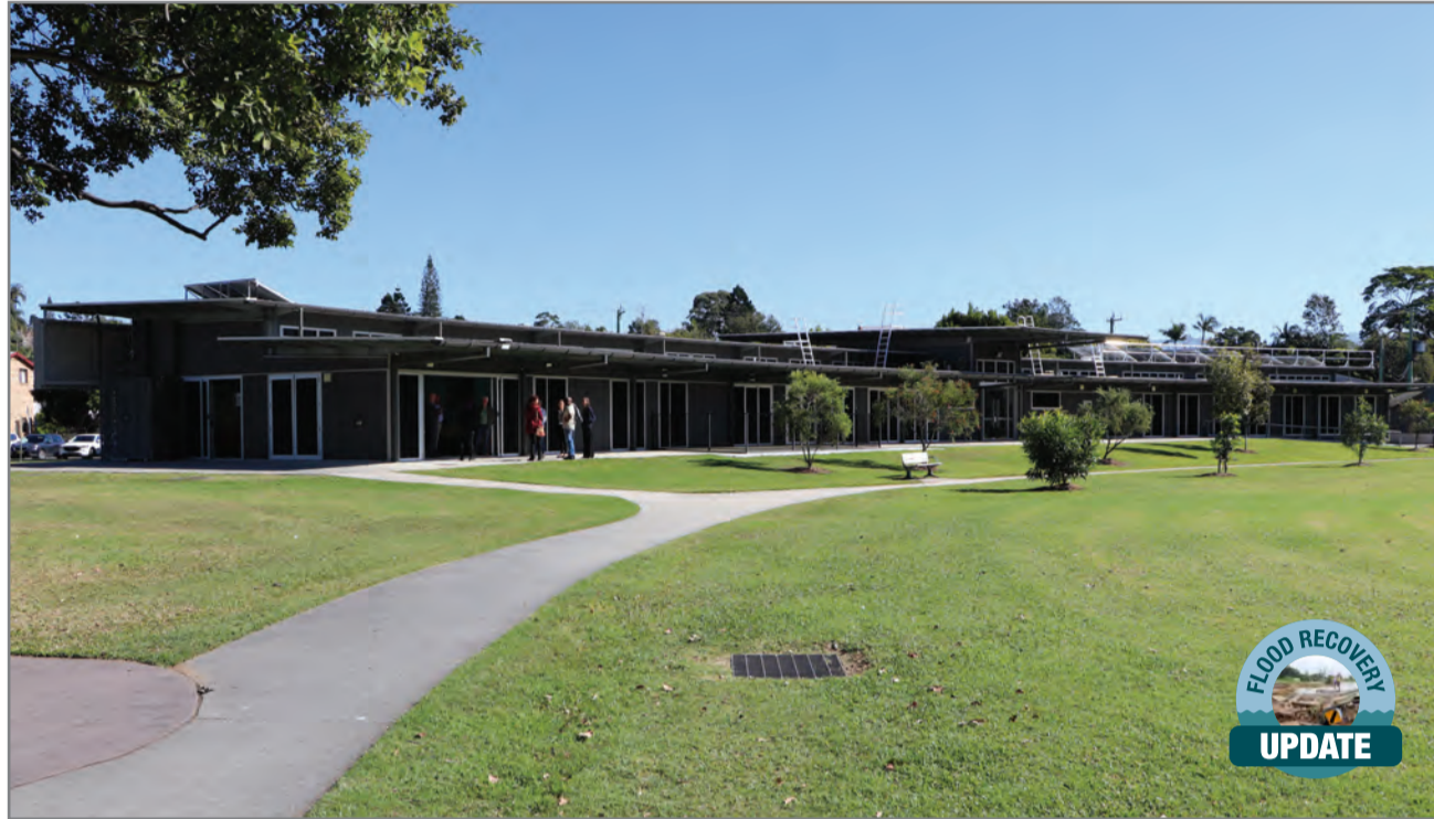
The Murwillumbah Community Centre in Knox Park is now back in operation following a significant restoration after damage from the devastating 2022 flood.
