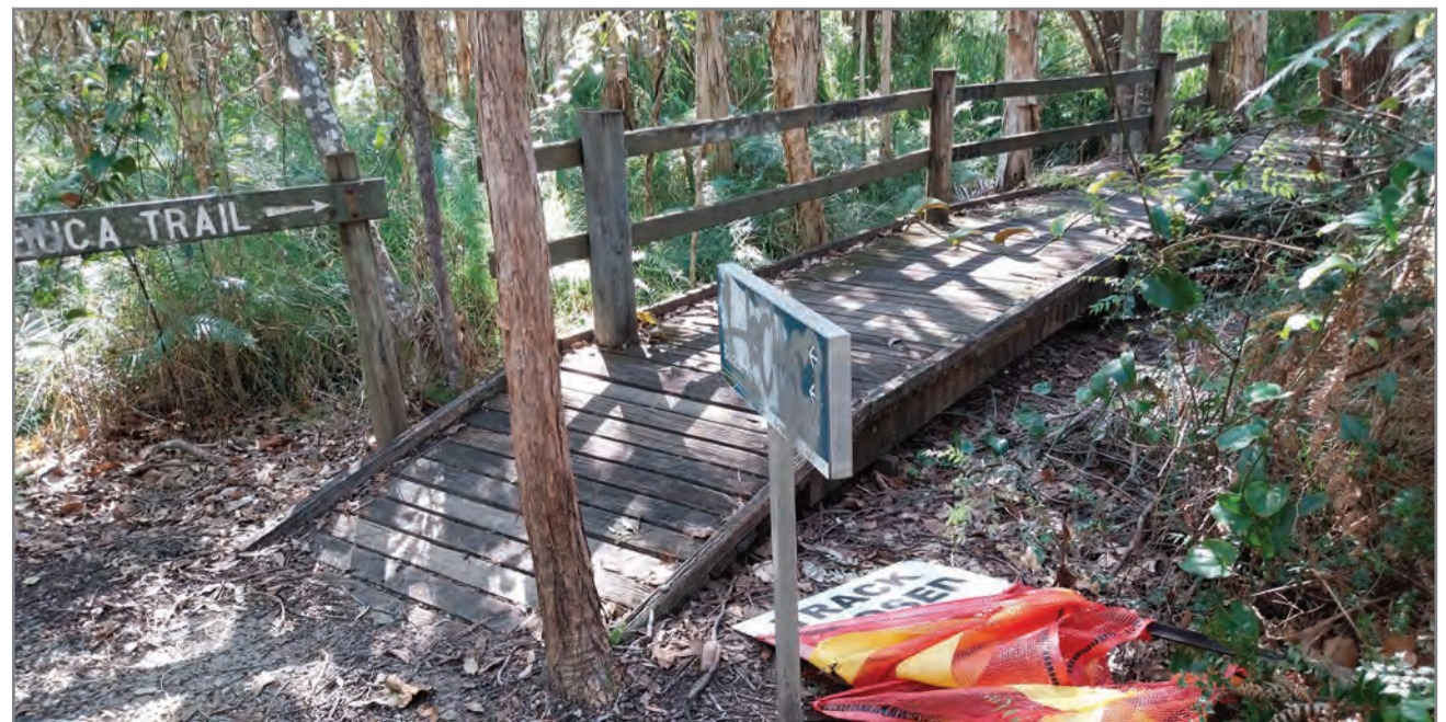
Vandals have removed 'tracks closed' signage and fencing numerous times at the Pottsville Environment Park, putting the community at risk.
