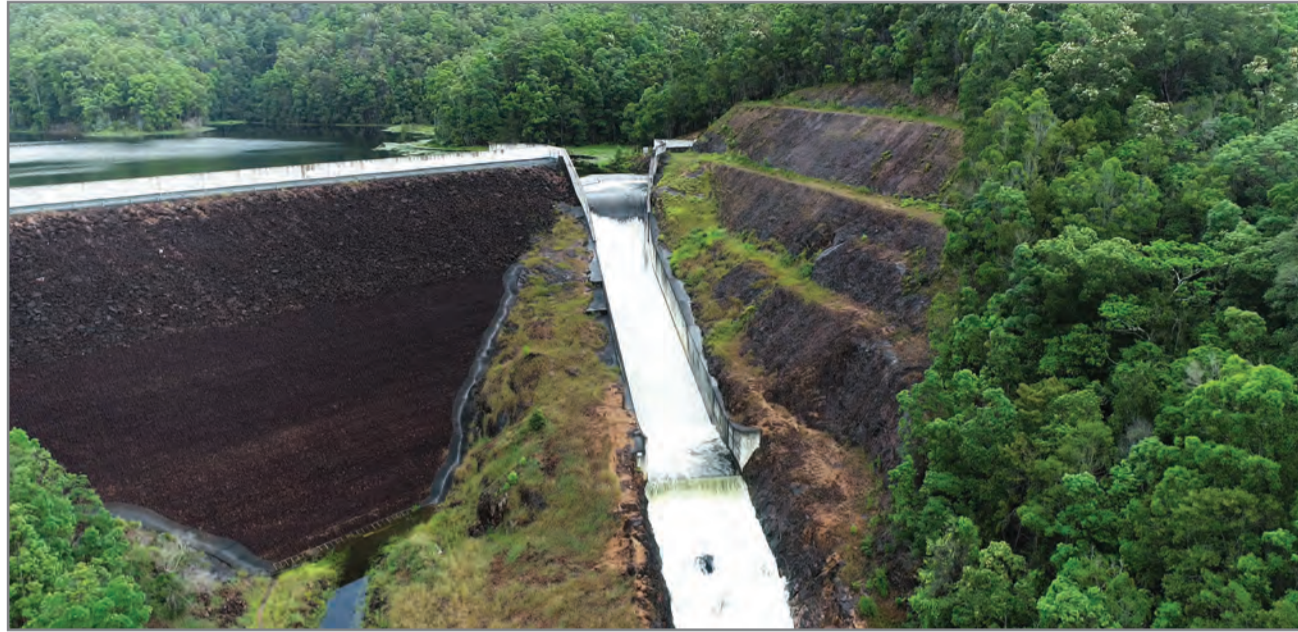
Under the proposal, the dam wall will rise by 8.5 metres, securing the Tweed's water supply until at least 2065.
