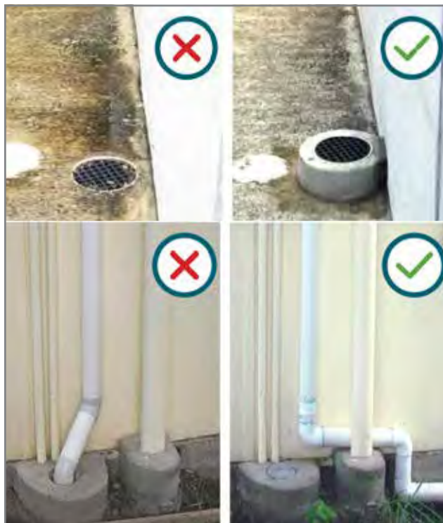
Top, make sure your overflow relief gully is compliant, and (above) check that your downpipes do not connect to your sewer pipes. Images courtesy of Unitywater.
