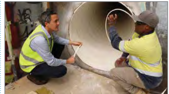
Council Flooding and Stormwater Engineer Leon McLean discusses the pipe relining process with Pipe Lining Pty Ltd's Jason Duval at the Lavender Creek pumping station site.
