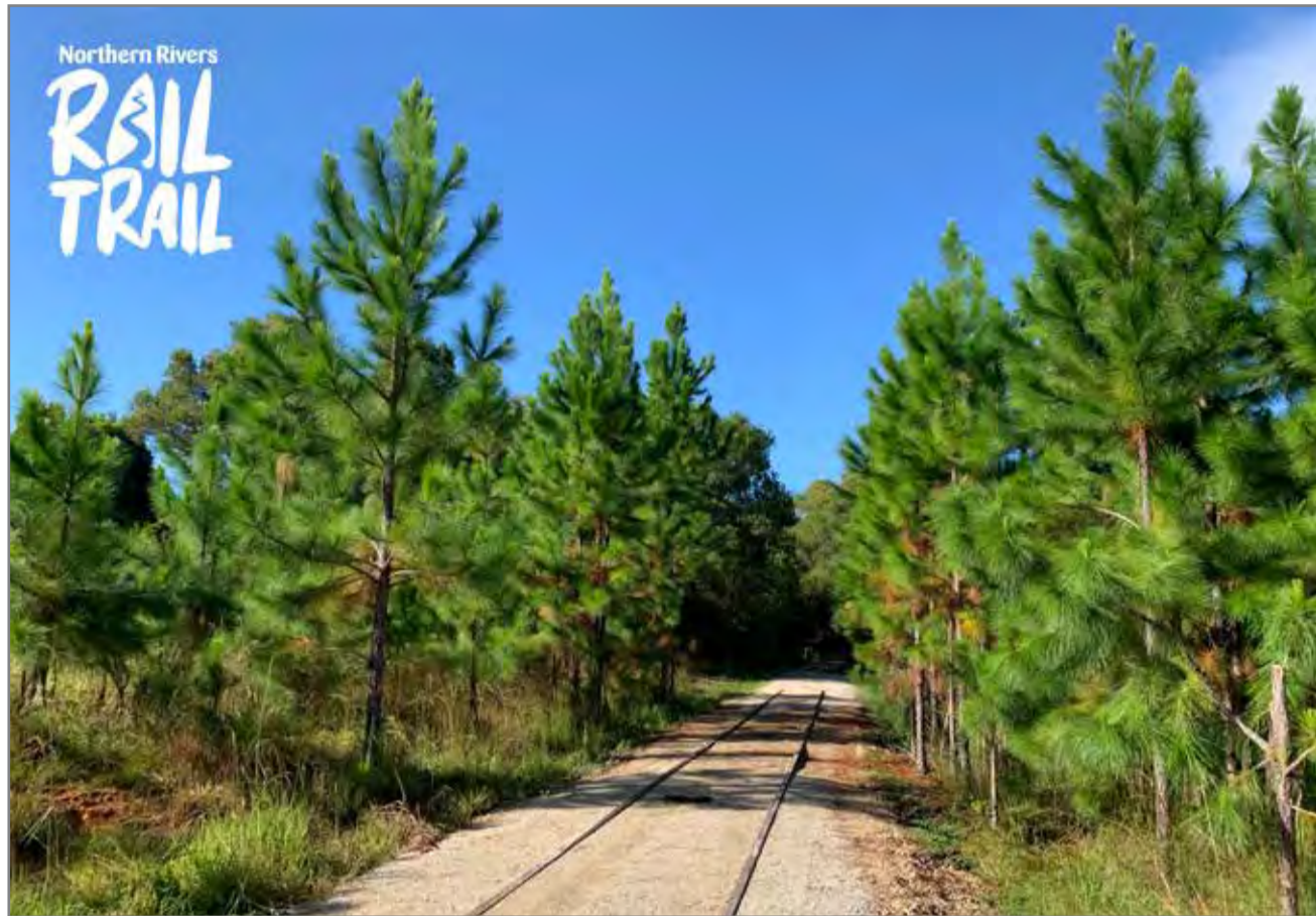
The trial surface near Stokers Siding along the Tweed section of the Northern Rivers Rail Trail withstood recent flooding events well. Compacted gravel, which is resistant to wet weather, will be used along much of the rail trail.
