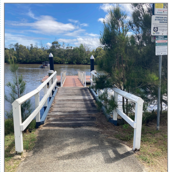
The current degraded jetty being repaired at Fingal New Boat Harbour.
