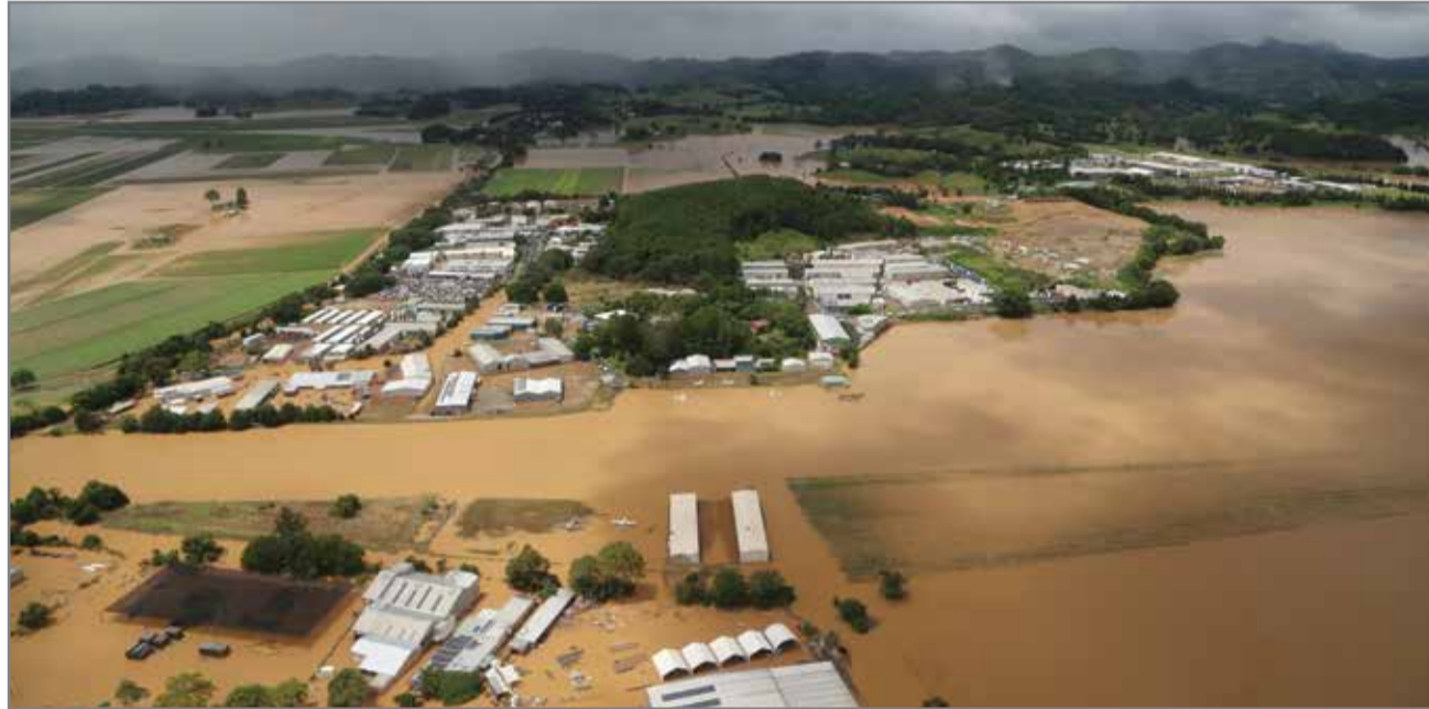
Floodwaters inundated much of the South Murwillumbah industrial area in the February 2022 flood.
