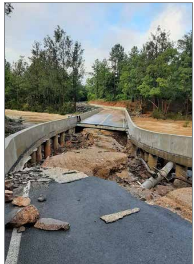
Byrill Creek bridge.
