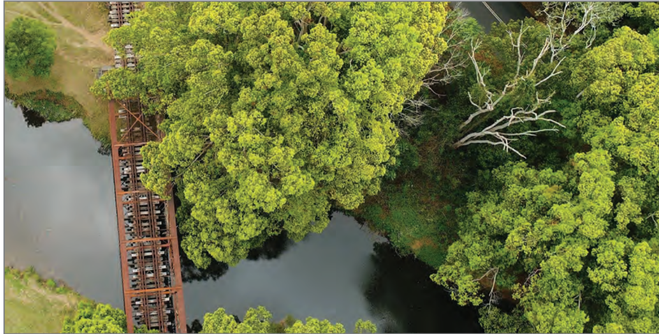
An aerial view of one of the bridges on the Murwillumbah to Crabbes Creek section of the proposed Northern Rivers Rail Trail.
