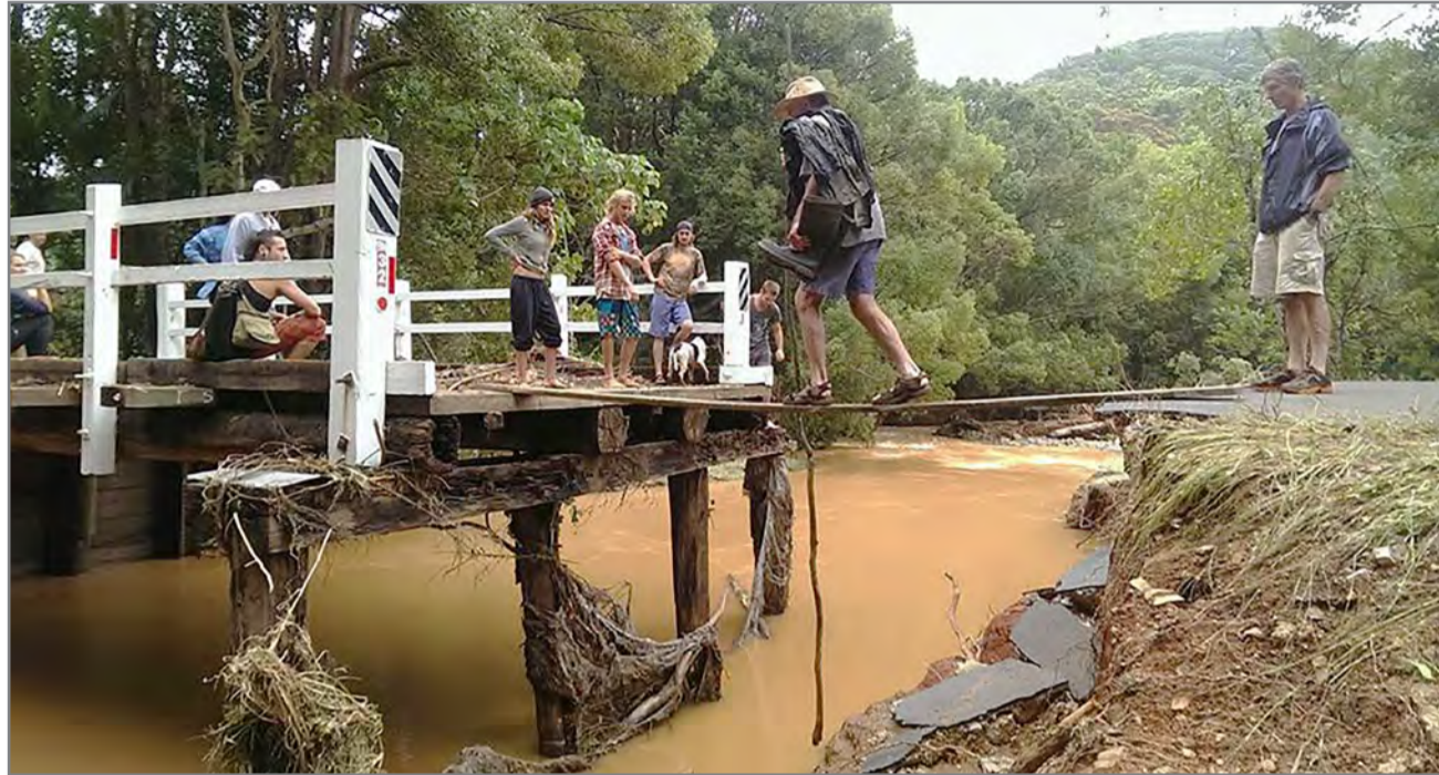
2017 flood damage to Shackells Bridge at Upper Burringbar. Photo: Serena V Dolinska
