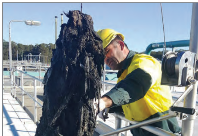
Pump assistant Craig Simpkins works to remove a mass of wet wipes and rags wrapped at the Banora Point Wastewater Treatment Plant.
