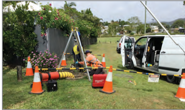
Contractors setting up flow gauges in Murwillumbah in 2018.
