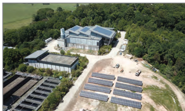
Under Council's Renewable Energy Action Plan, Council has completed a range of energy efficiency works, including this solar installation at Bray Park Water Treatment Plant.
