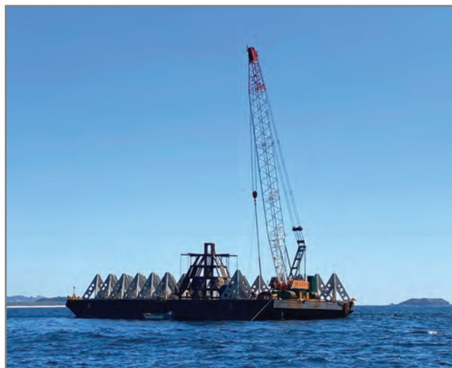
The new $1 million artificial reef being installed off the Tweed Coast.
