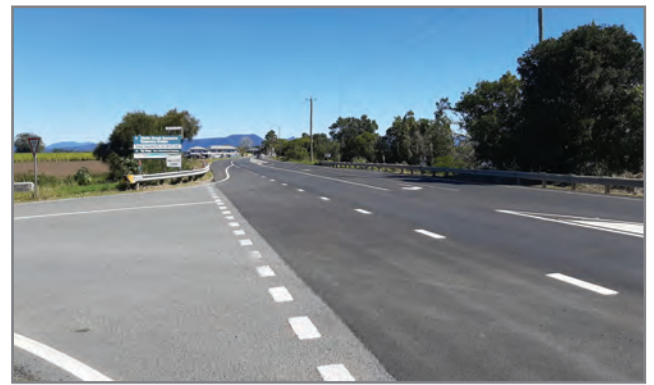
The upgraded intersection on Tweed Valley Way at Bartletts Road.
