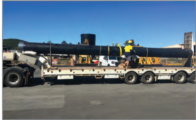
The pipe is loaded for delivery to site.
