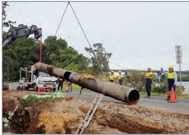
The old pipe is lifted from the trench.
