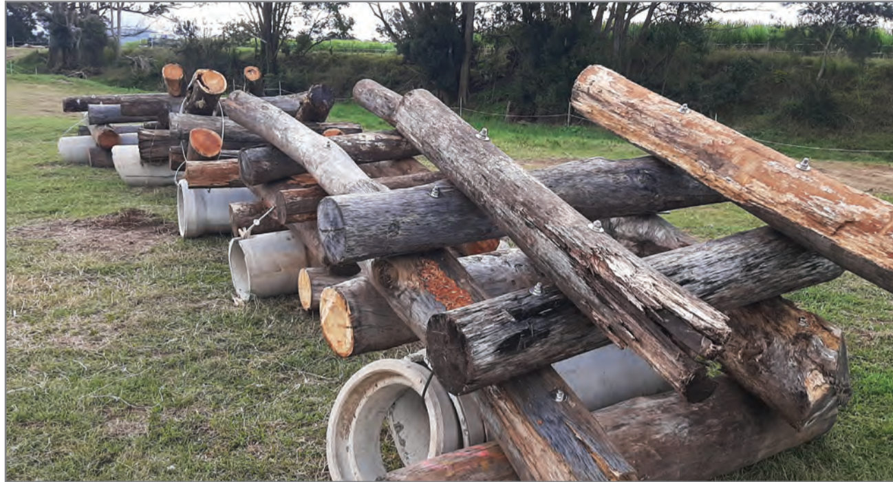
The five fish hotels installed in the Tweed River near Dunbible Creek. The hotels replicate naturally occurring snags.
