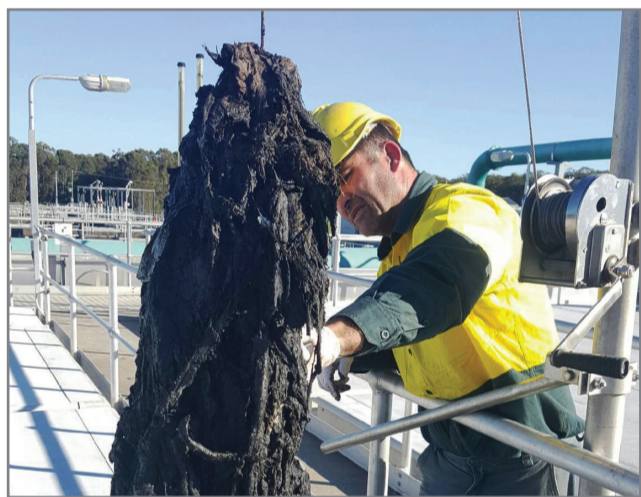
A worker lifts a pump at the Banora Point Wastewater Treatment Plant covered in a mess of wet wipes and other non-flushables.
