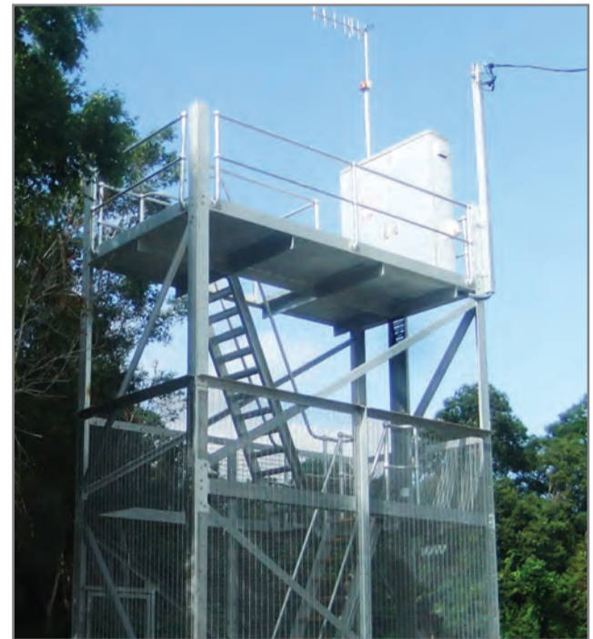
Raised pump station platform on Tree Street, Bray Park.
