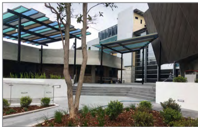
The Tweed Heads Civic and Cultural Centre redevelopment is nearing completion.
