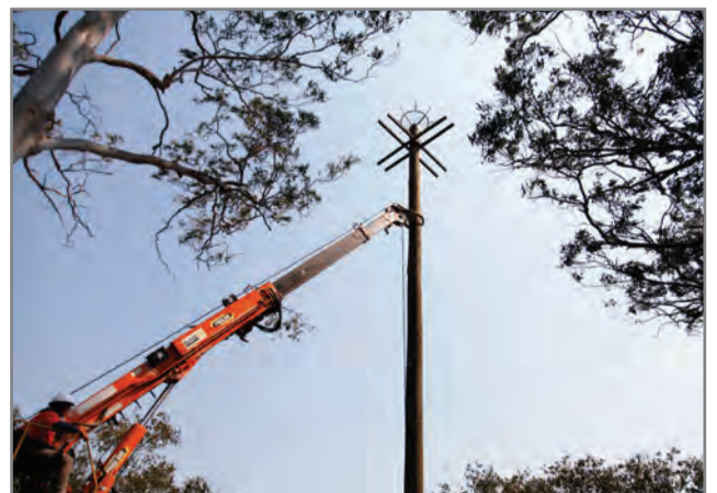
The new osprey nesting cradle being craned into position.
