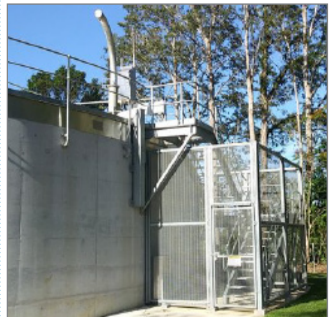
The new Chamber reservoir will provide additional water supply for the Terranora area.
