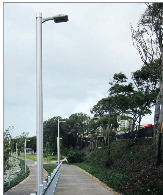
An example of the light poles to be installed from Cathedral Court south to Dryandras Court.
