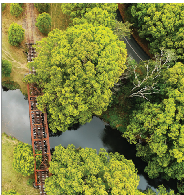
A bridge in Stokers Siding – one of 18 historic bridges along the proposed rail trail route.
