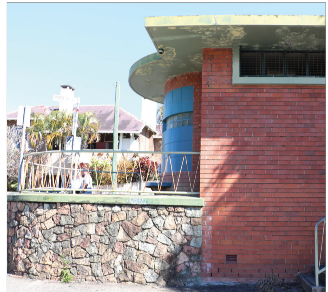
There's life in this old amenities block yet, with a restoration of its heritage features ahead and hopefully a new future as a community space.
