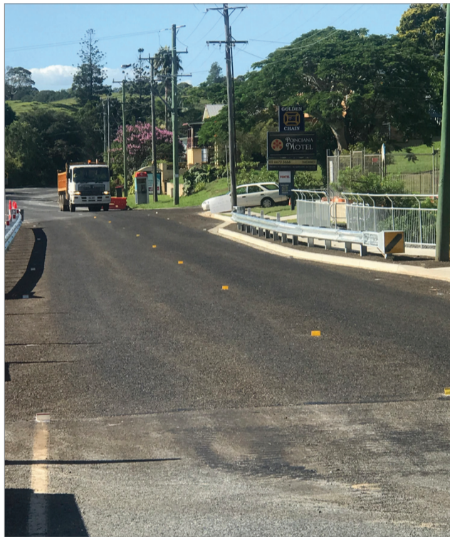
Tweed Valley Way at Blacks Drain, South Murwillumbah, now open to traffic.
