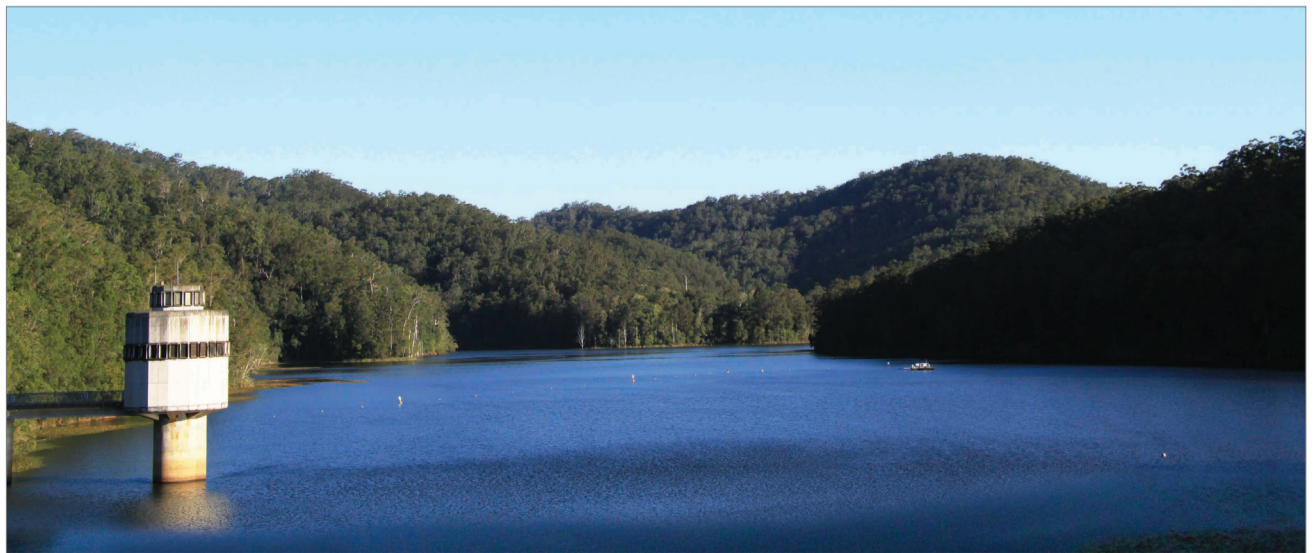
The capacity of Clarrie Hall Dam will treble once the dam wall has been raised, securing Tweed’s water supply into the future.
