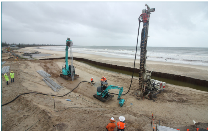
Piling works on the southern end of the site.
