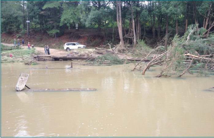
Where Byrrill Creek Bridge used to be.
