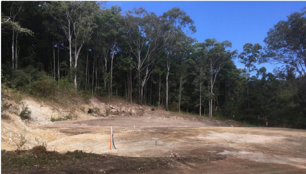
Image: Pottsville koala holding facility site pad ready for construction September 2020
