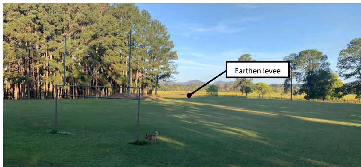
Plate 3 View looking south-east showing Murwillumbah High School sports field in foreground and earthen levee in background
