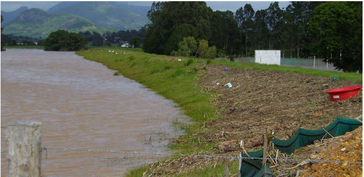
Plate 1 View of earthen levee looking west from Commercial Road taken after the peak of the March 2017 flood (note flood debris at crest of levee)
