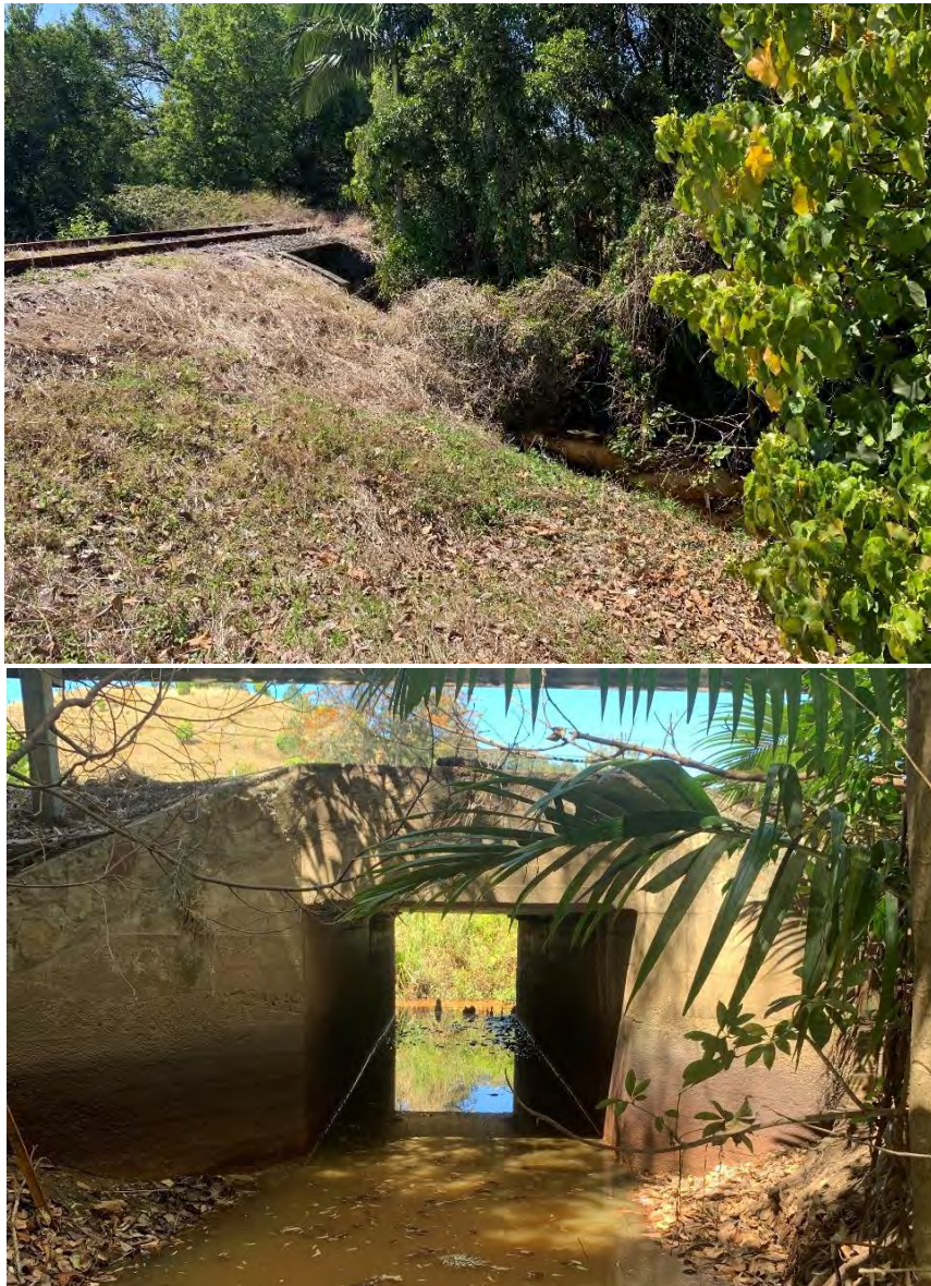
Figure 3-1: Top: Railway culvert, bottom: Road culvert
